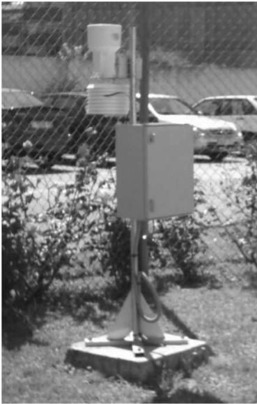
Figure 4: Final assembly and WS installation.
