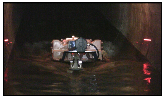
Figure 1: The cable-guided damage surveying system within a sewer pipe.
