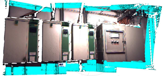
Figure 4: 3D model of a room reconstructed from several colored time-of-flight images. The surface of 3D measurements for which no color is available is colored in blue.
