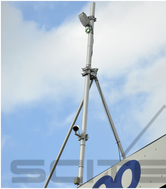
Figure 2: ZXY radio receiver mounted on antennas around the stadium.
