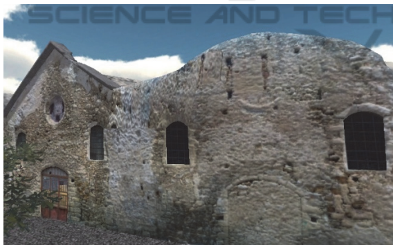
Figure 12: Currently, there is a missing part on top of the building.
