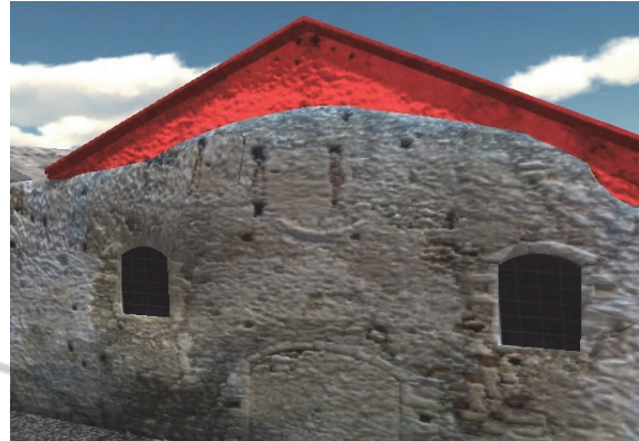
Figure 13: Digital restoration of the missing part; the red part does not exist at present.
