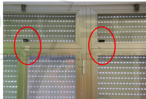
Figure 1: Magnetic sensors for windows opening detection.
