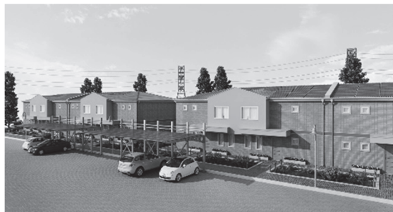
Figure 8: Buildings and car parks in demo site.
