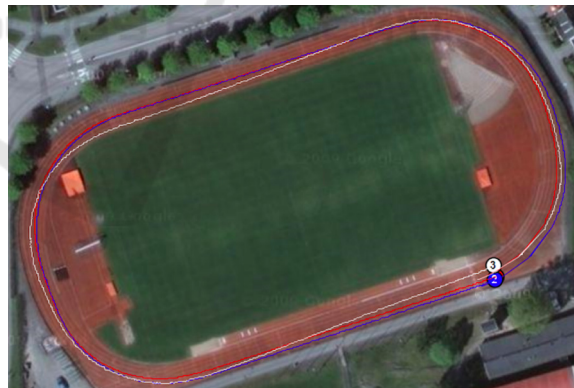
Figure 6: Measurements from Vallhamra sports facilities.
