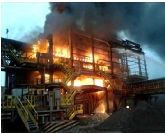
Figure 3: Fire on belt conveyor system TR-315K-36.
