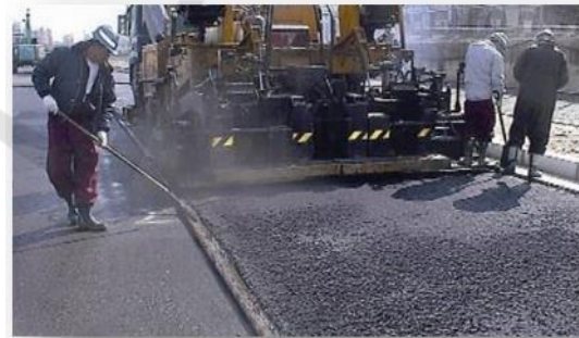
Figure 5: The utilization of Waste Ore into Asphalt Material.
