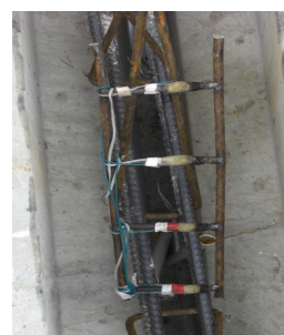
Figure 5 site buried seam strain measurement point
