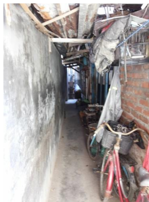
Figure 1: Inadequate evacuation route.
