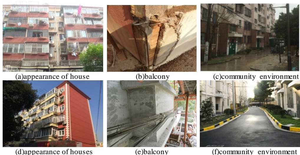
Figure 2. Comparison between before and after retrofit of sound insulation renovation.
