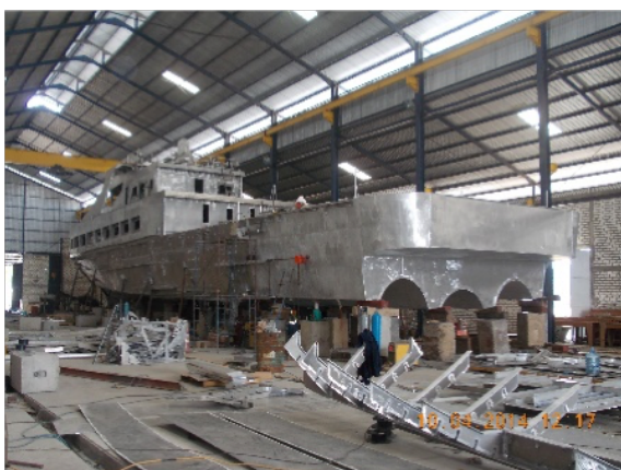
Figure 1: A Hard-chine Crew Boat during The Production Process (courtesy of PT. Orela Shipyard).
