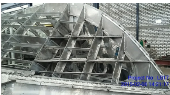
Figure 2: Construction Part of The Hard-chine Orela Crew Boat Near The bow (courtesy of PT. Orela Shipyard).
