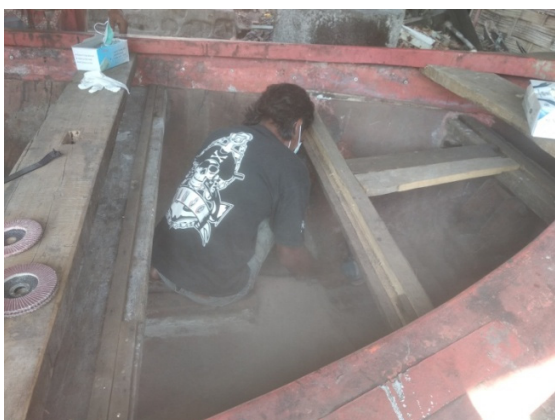
Figure 3: Cleaning of the hull before the repair process.
