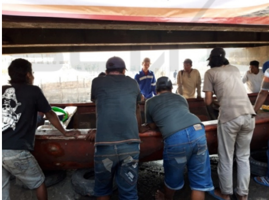
Figure 2: Briefing of participants before the repair process.
