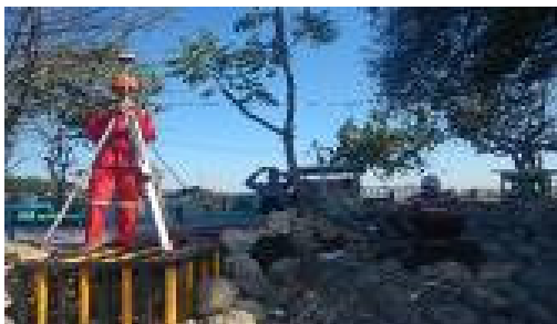
Figure 4: Determine Point Control.
