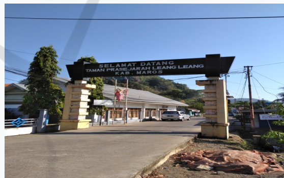
Figure 3: The area gate looks stiff and formal like a factory area (Source: R. CecepEkapermana).
