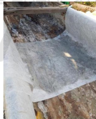
Figure 12: Installation of fiberglass fiber.
