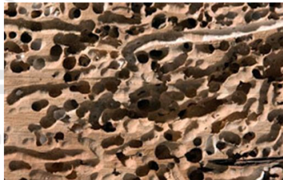
Figure 3: Leakage because of sea animals.
