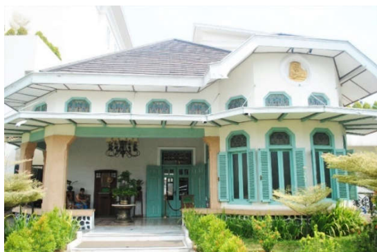
Figure 5: The Peranakan style façade of The Sidji Hotel (Budianto, 2018).
