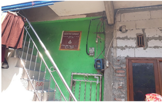
Figure 1: Condition of the Kapuas alternative school in Putat Jaya Village
