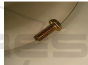
Figure 3. Suspension defect on the ground side in GIS.
