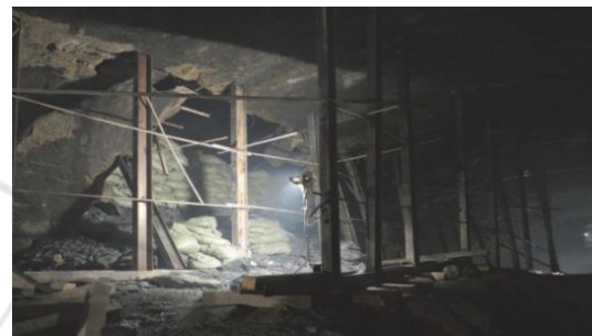
Figure 3: Collapse due to a fractured zone.
