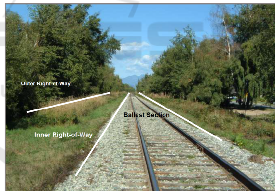
Figure 1: Different zones on and around the rail tracks where vegetation management is needed. Image source CN (2019).
