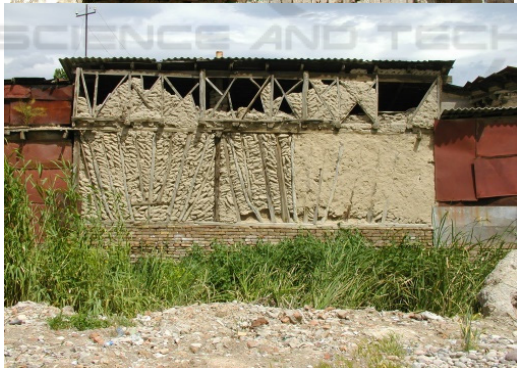
Figure 5: Incomplete houses with wooden frame filled with air bricks or guvala (“sinch”) (photo by P. Burton).
