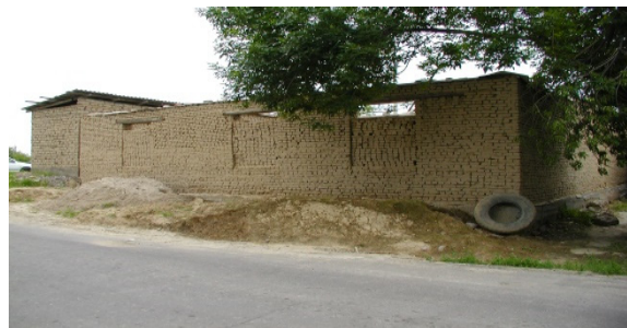
Figure 4: Incomplete houses from air bricks (photo by P. Burton).
