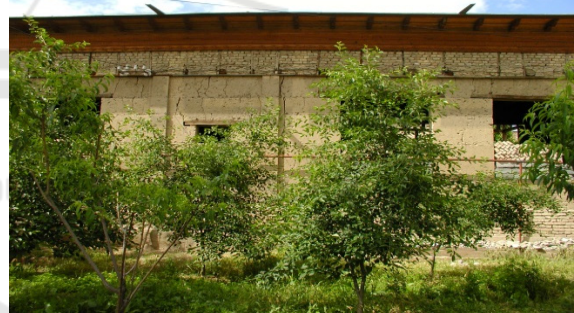
Figure 3: Incomplete houses from loam and bricks (photo by P. Burton).
