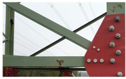
Figure 5: In this image, three corrosion damages from other pictures have been pasted onto undamaged components using the Poisson Image Editing (Pérez et al., 2003) technique.
