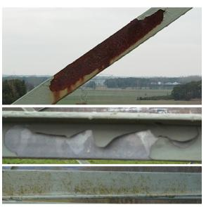
Figure 1: Examples of a corrosion damage, a missing painting damage and a patch of dirt, from top to bottom.
